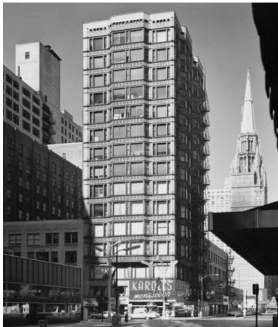
Fig. 17.38 El Reliance Building de Chicago.
