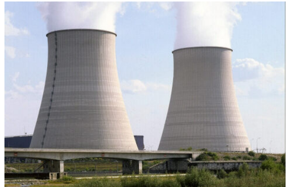
Fig. 21.3 Le torri evaporative.
