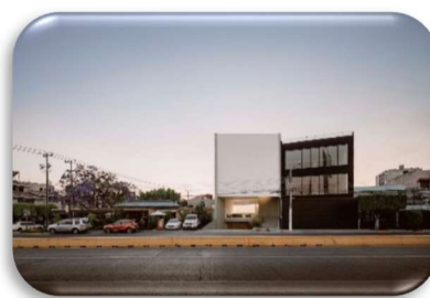
XIII. Fachada Archdaily.
