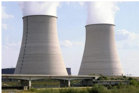
Fig. 21.3 Le torri evaporative.
