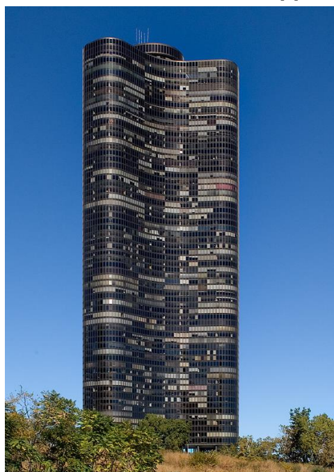
Fig. 20.13 Lake Point Tower a Chicago.
