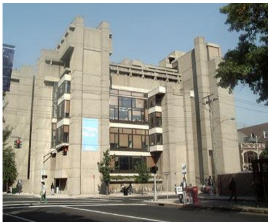
Fig. 19.35 Art and Architectural Building (New Haven).
