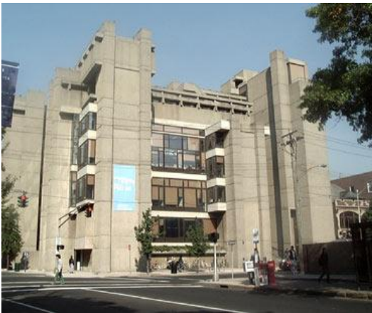
Fig. 19.35 Art and Architectural Building (New Haven).
