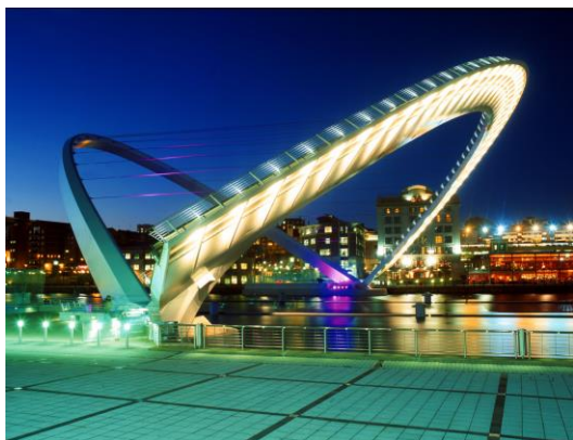
Fig. 21.5 Il Thyne Millennium Bridge a Gateshead (Chris Wilkinson).
