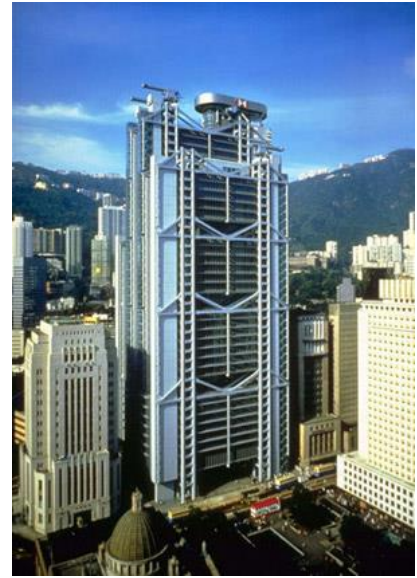
Fig. 20.19 La Hong Kong & Shanghai Banking Corporation.
